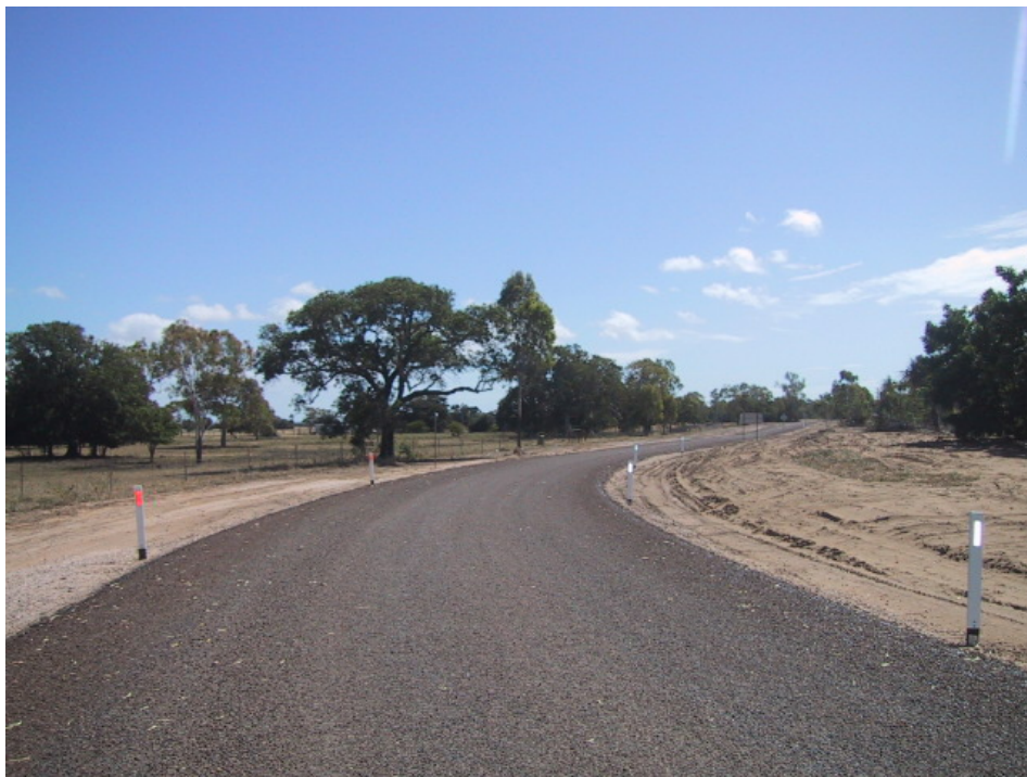
Sandhills Road (bitumen construction)
