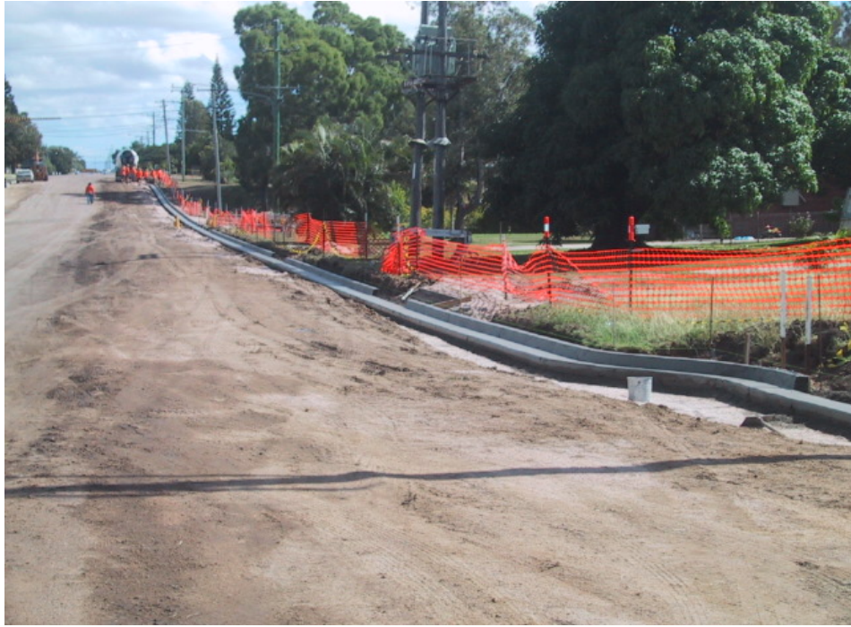
Chippendale Street (kerb and channel works)
