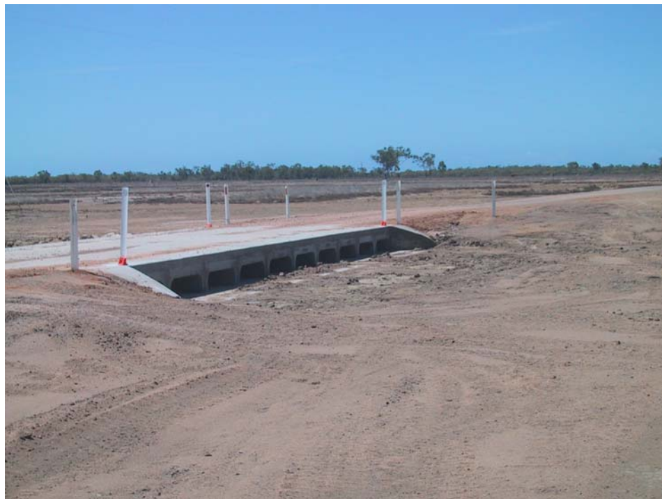
Jerona Road (drainage works)
