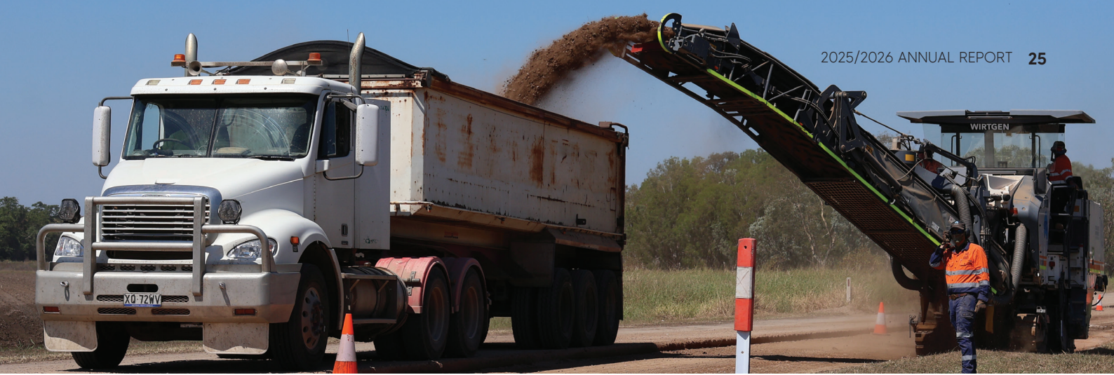
📍 Bahr Road, Giru Road Works
