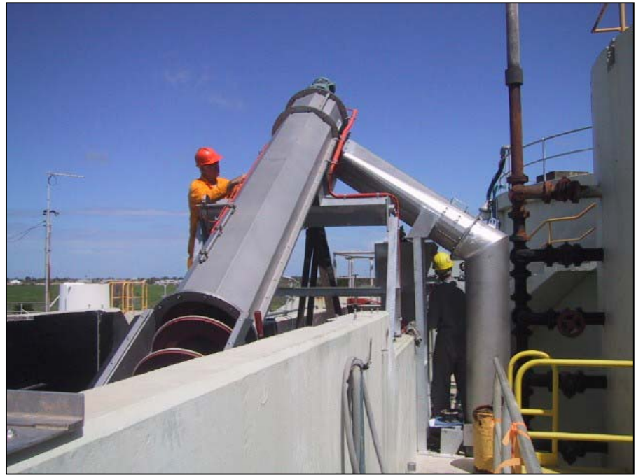
Installation of mechanical inlet screen at Ayr Sewerage Treatment Plant
