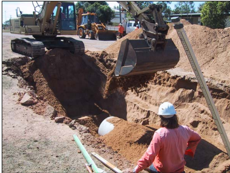
Henry Street during construction
