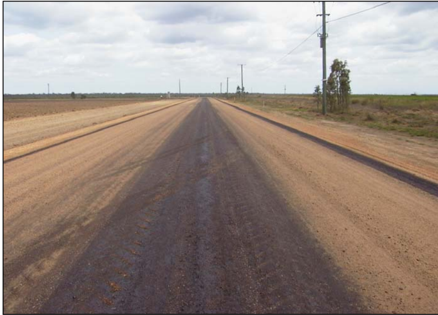
Construction of Day Road
