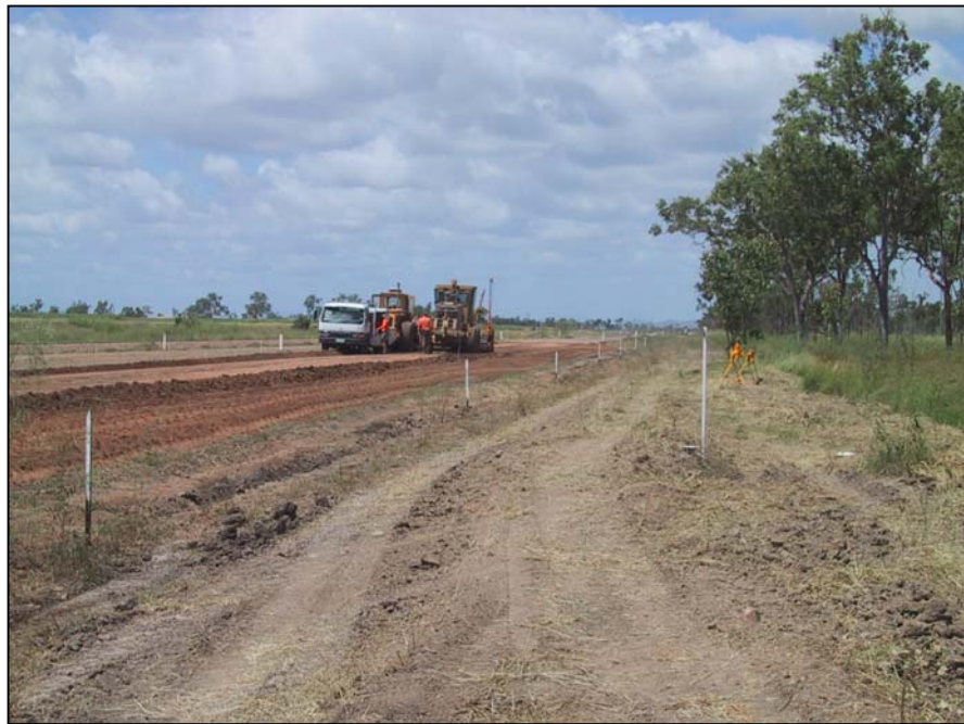
Barratta Road construction
