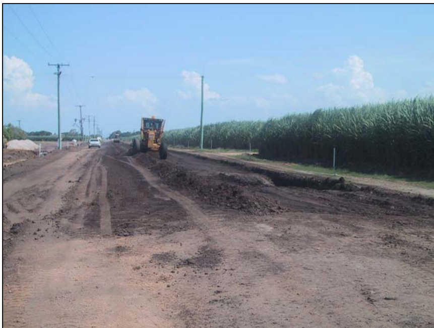
Colevale Road construction
