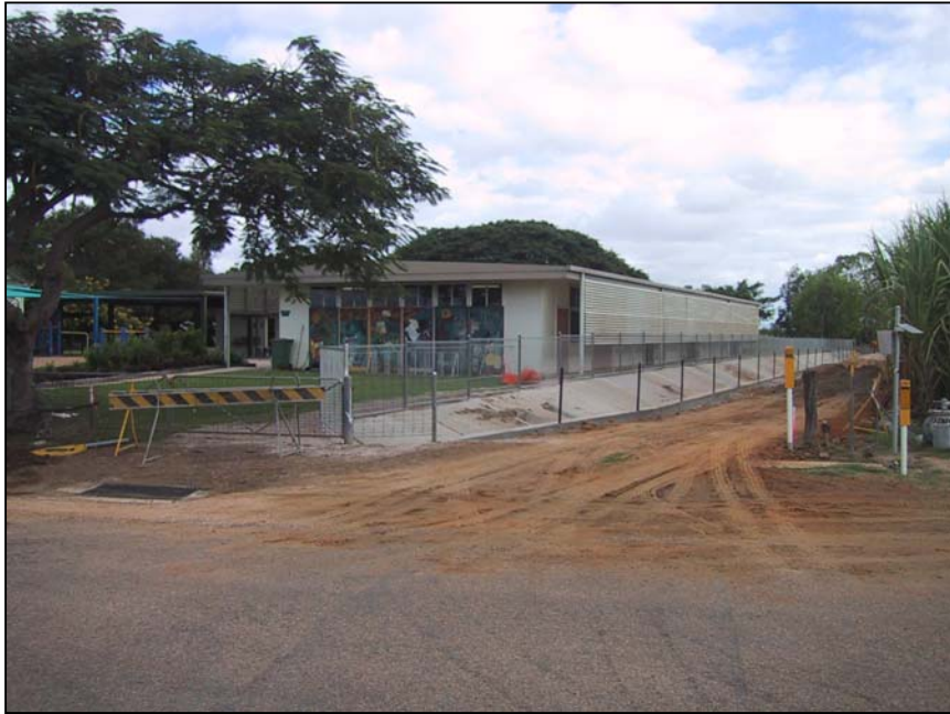
Clare School drainage and footpath
