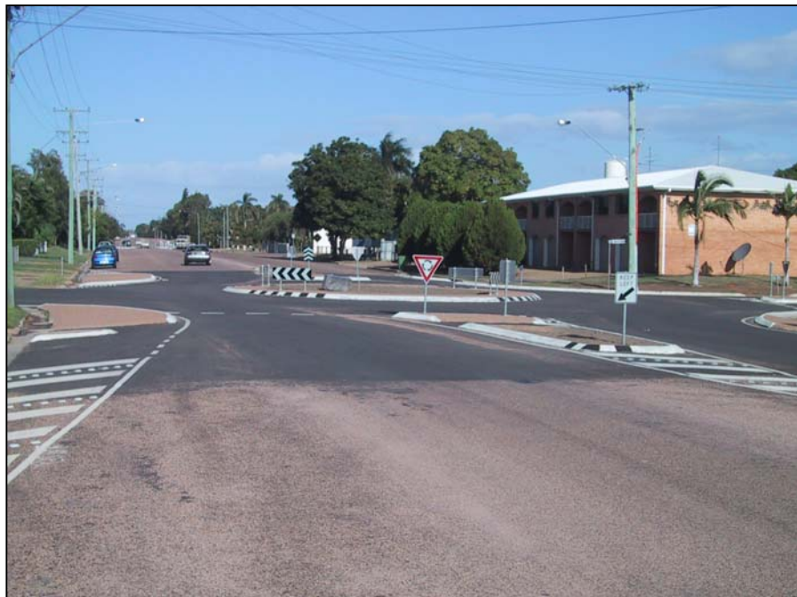
Cox Street / Chippendale Street Roundabout
