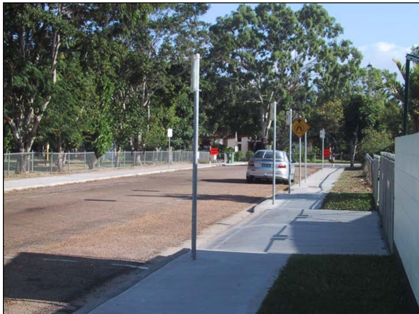
Davenport Street Footpath
