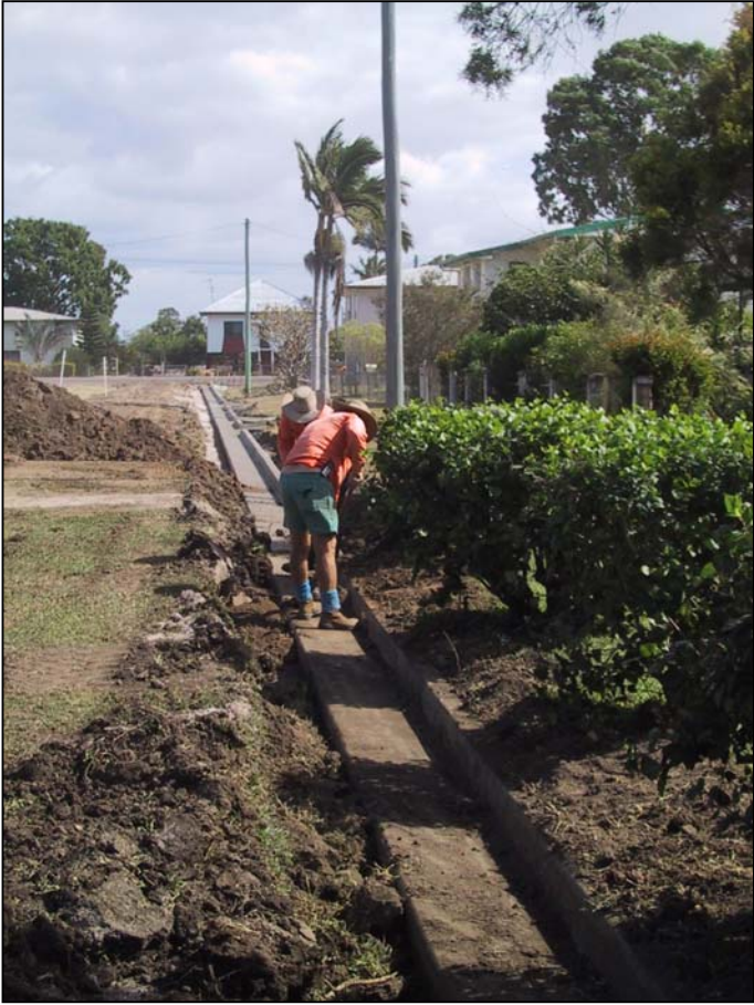
Third Street kerb and channel
