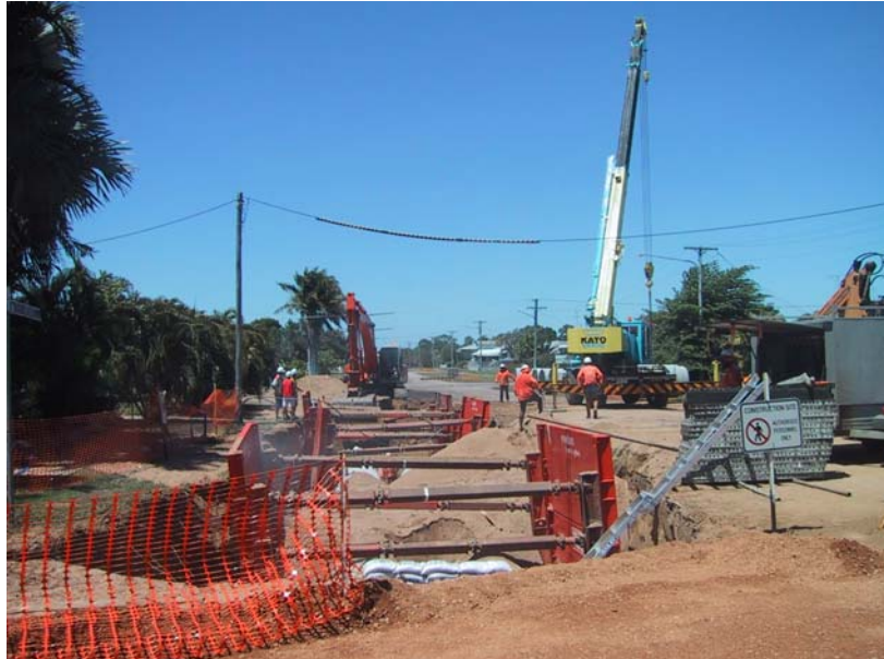
Construction of 12 th Avenue Drainage Scheme in Home Hill.
