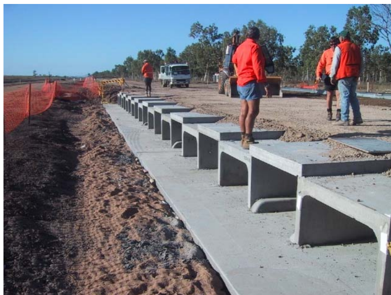
Bitumen Construction of Barratta Road
