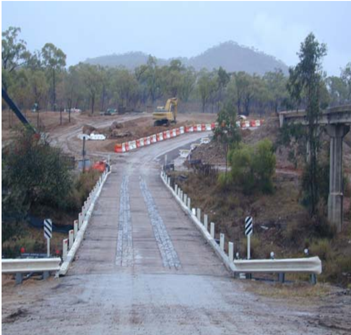
Ongoing Construction on the Expedition Pass Creek Bridge near Dalbeg.
