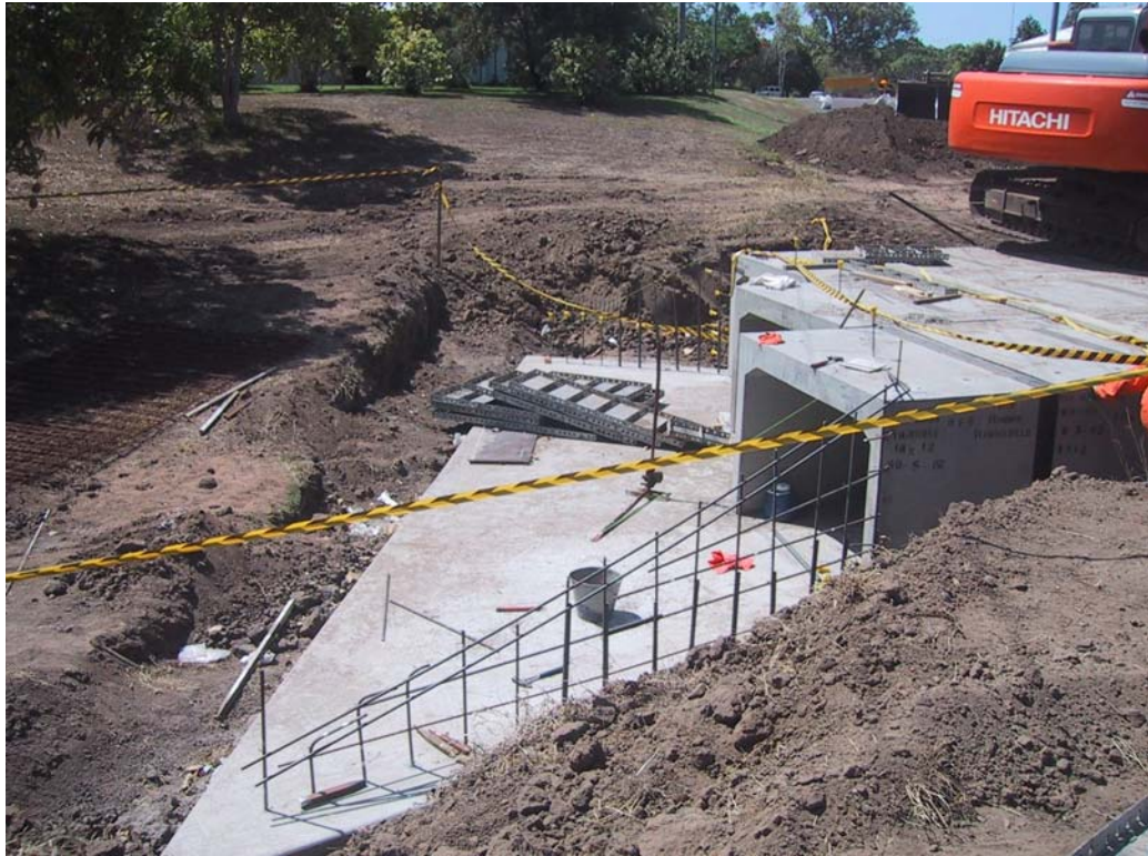
Drainage Works in Kidby Gully, Home Hill
