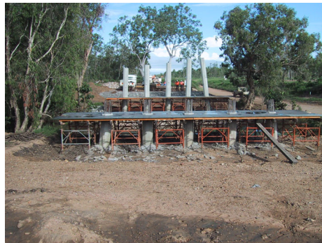
Barratta Bridge during construction
