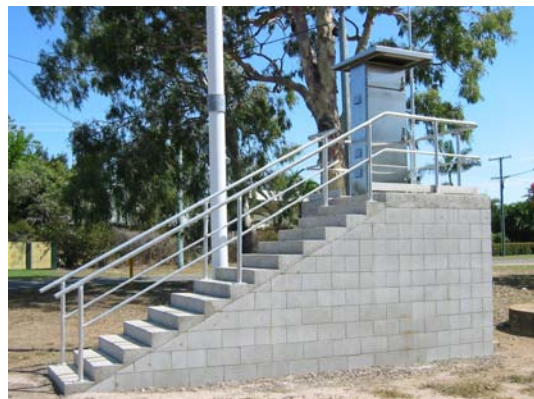
Sewerage Switchboard Replacement, Nelson's Lagoon, Ayr
