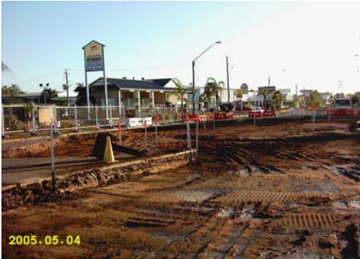
Construction of Roundabout, Queen and Little Drysdale Street, Ayr
