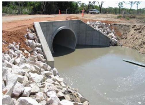
Completed upgrade of drainage, Groper Creek Road
