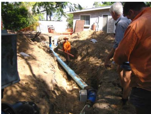
Installation of new pipe work for Bore 15, Ayr
