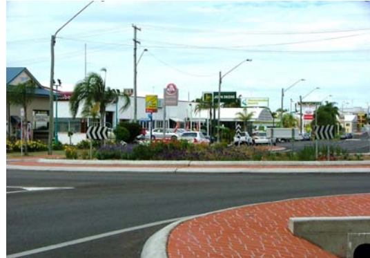
Completed Roundabout, Queen and Little Drysdale Street, Ayr
