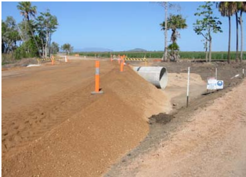
Upgrade of road and drainage, Groper Creek Road
