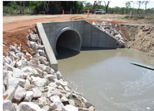
Completed upgrade of drainage, Groper Creek Road
