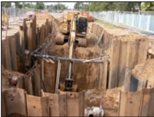
Council work men reconstructing failed sewerage manhole in Chippendale Street, Ayr
