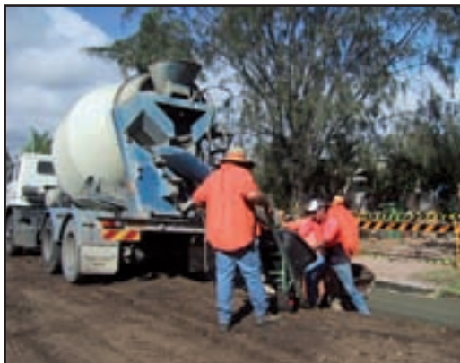
Construction of kerbing and channelling in Braby Street, Alva Beach
