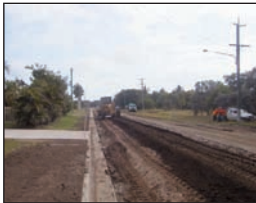
Road construction of Braby Street, Alva Beach
