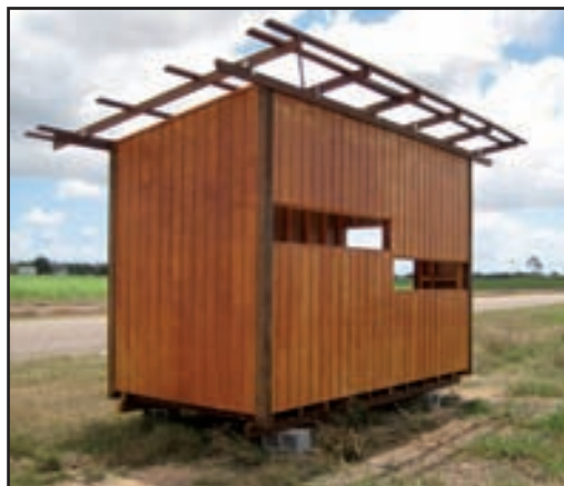
Partially constructed bird hide on Hodel Road, Giru
