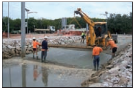
Council constructing pontoon at Plantation Creek
