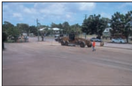
Council constructing new carpark as contractor for Ayr Golf Club
