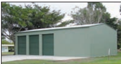
Clare Co-locate facility - Headquarters building for Clare State Emergency Service & Clare Rural Fire Brigade
