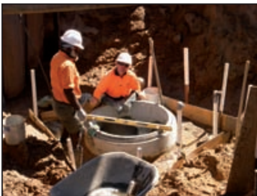
Repair works to sewerage lines in Chippendale Street, Ayr
