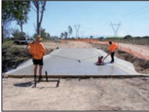
Reconstruction of concrete floodway on Woodhouse Road (near Gladys Lagoon)
