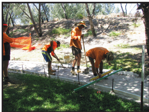
Council workers constructing pathway at Alva.
