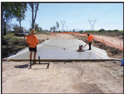
Construction of concrete floodway on Woodhouse Road (near Gladys Lagoon)
