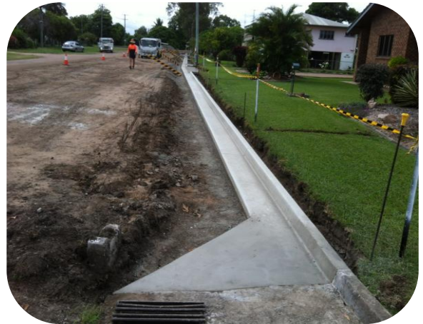
New Kerbing & Channelling in Thirteenth Avenue Home Hill
