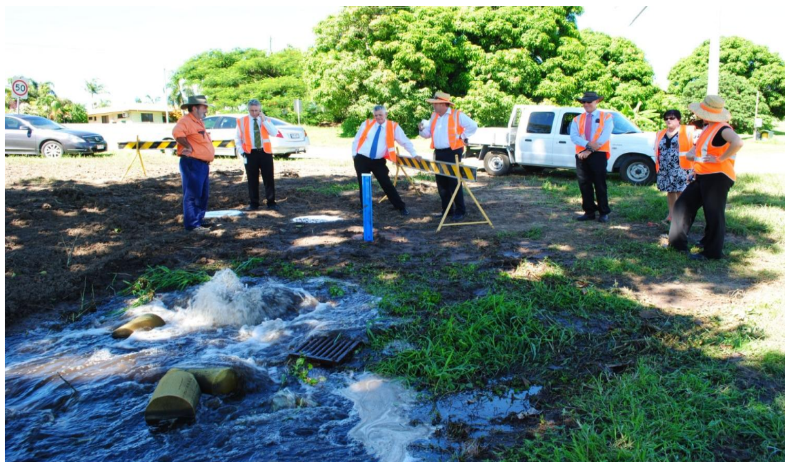
(Above) Scouring 250 mm Water Main from South Ayr to Rossiters Hill Ayr
