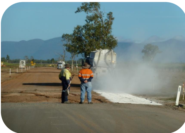
Sayers Road, Barratta - Lime Stabilisation of subgrade prior to bitumen construction
