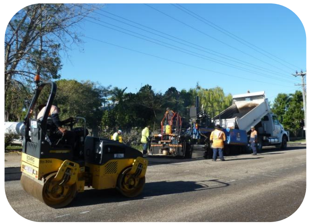
Laying Asphalt in Burke Street Ayr
