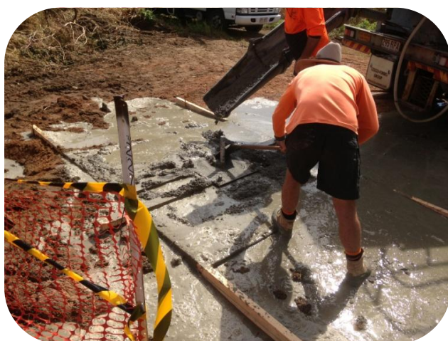
Constructing concrete foundations for new Flood Reporting Station at Yellow Gin Creek
