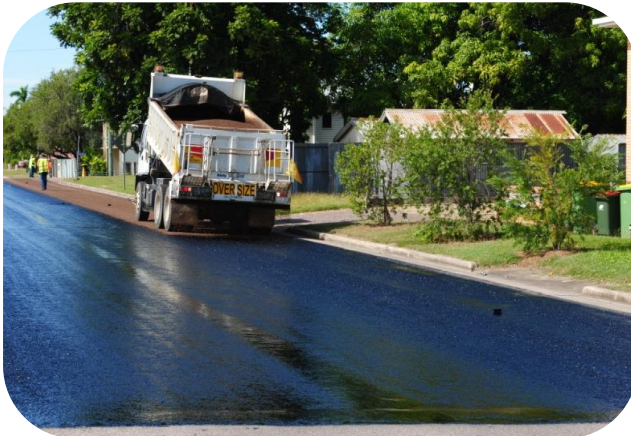
Bitumen Resealing works in Chippendale Street, Ayr
