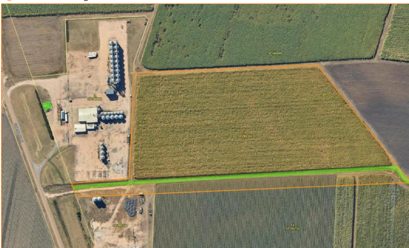
Figure 3: Aerial image of Lot 10 on SP289356
