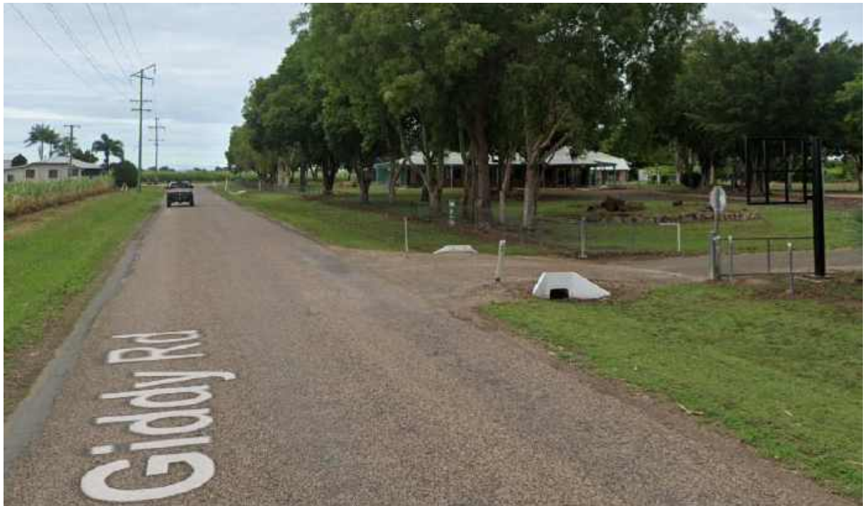
Figure 5.4 – Giddy Road table drain and culverts (Google Maps)
