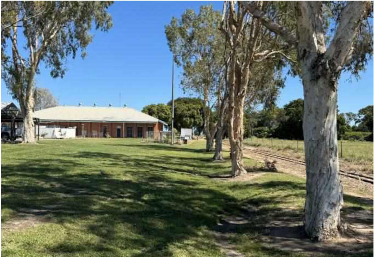
Figure 5.5 – Existing open drain between subject site and tram line (site photo)
