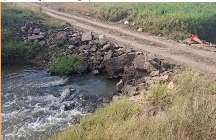
Figure 5: Existing culvert crossing to proposed Lot 4
