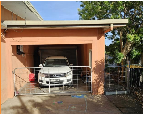
Figure 3: Open carport - Dwelling house on Lot 4
